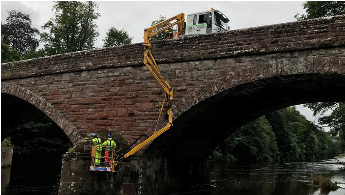
Figure 14 - Underbridge Access Unit
